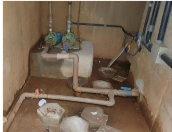
*Foto 10 – Bombas de recalque*
