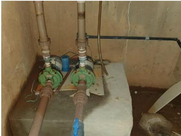
*Foto 09 – Bombas de recalque*
